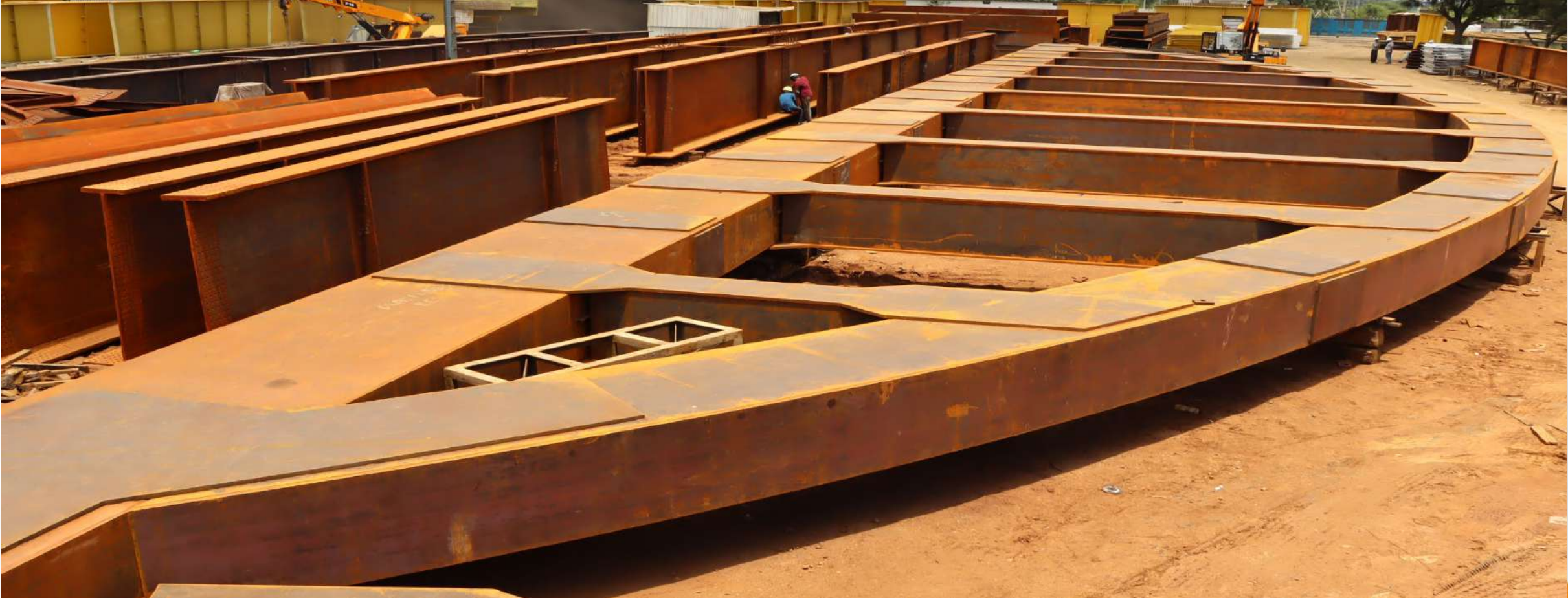
ONE SIDE ARCH OF 54.0M SPAN BOW STRING GIRDER – RAIGNAJ – DRAIPL
