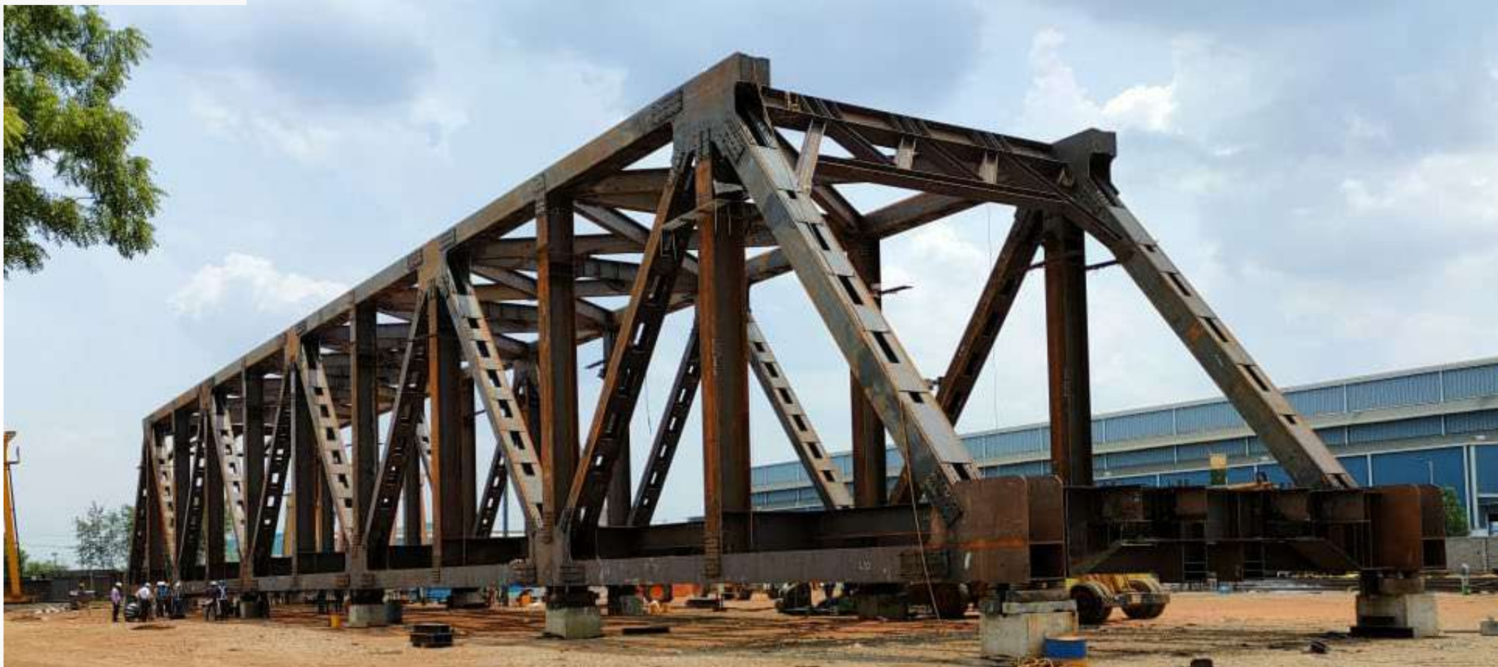
79.0M SPAN OPEN WEB GIRDER – PUNE METRO - NCC
