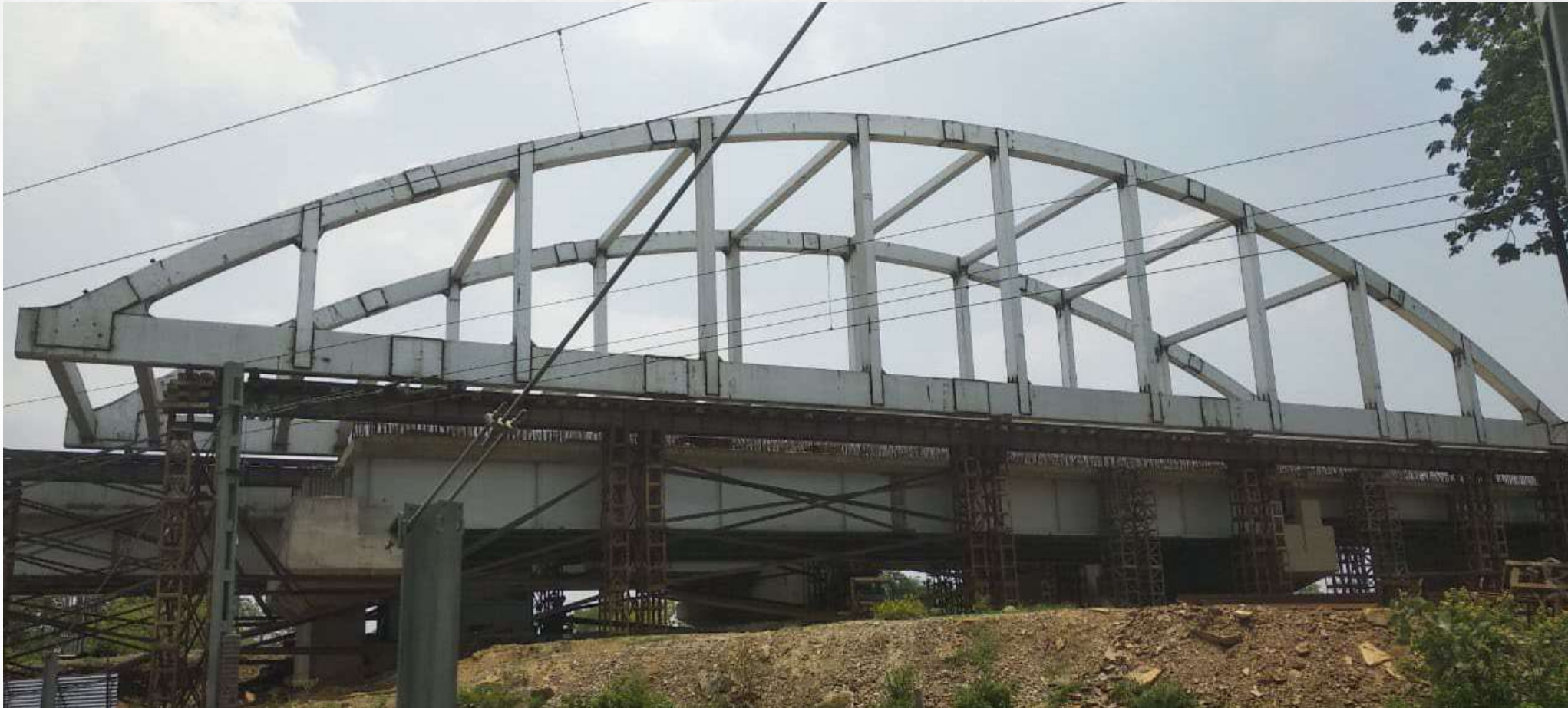
60.0M BOW STRING GIRDER – JHARKHAND
