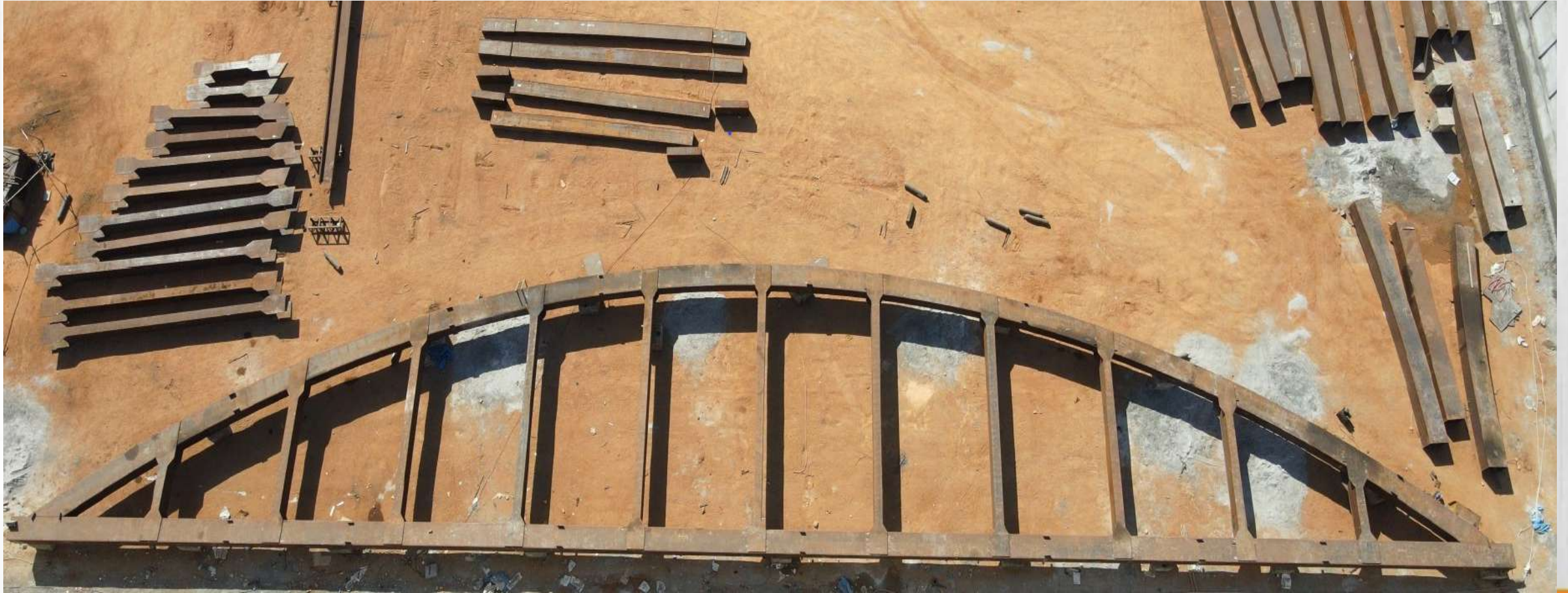
ONE SIDE ARCH OF 72.0M SPAN BOW STRING GIRDER – NAGPUR - MRIDC
