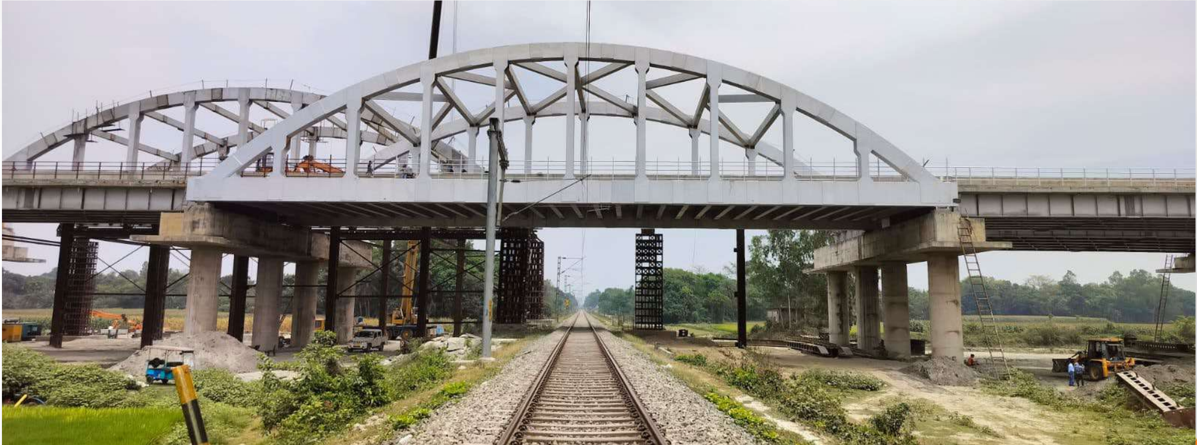
48.10M CLEAR SPAN BOW STRING GIRDER – RAIGANJ, WEST BENGAL
