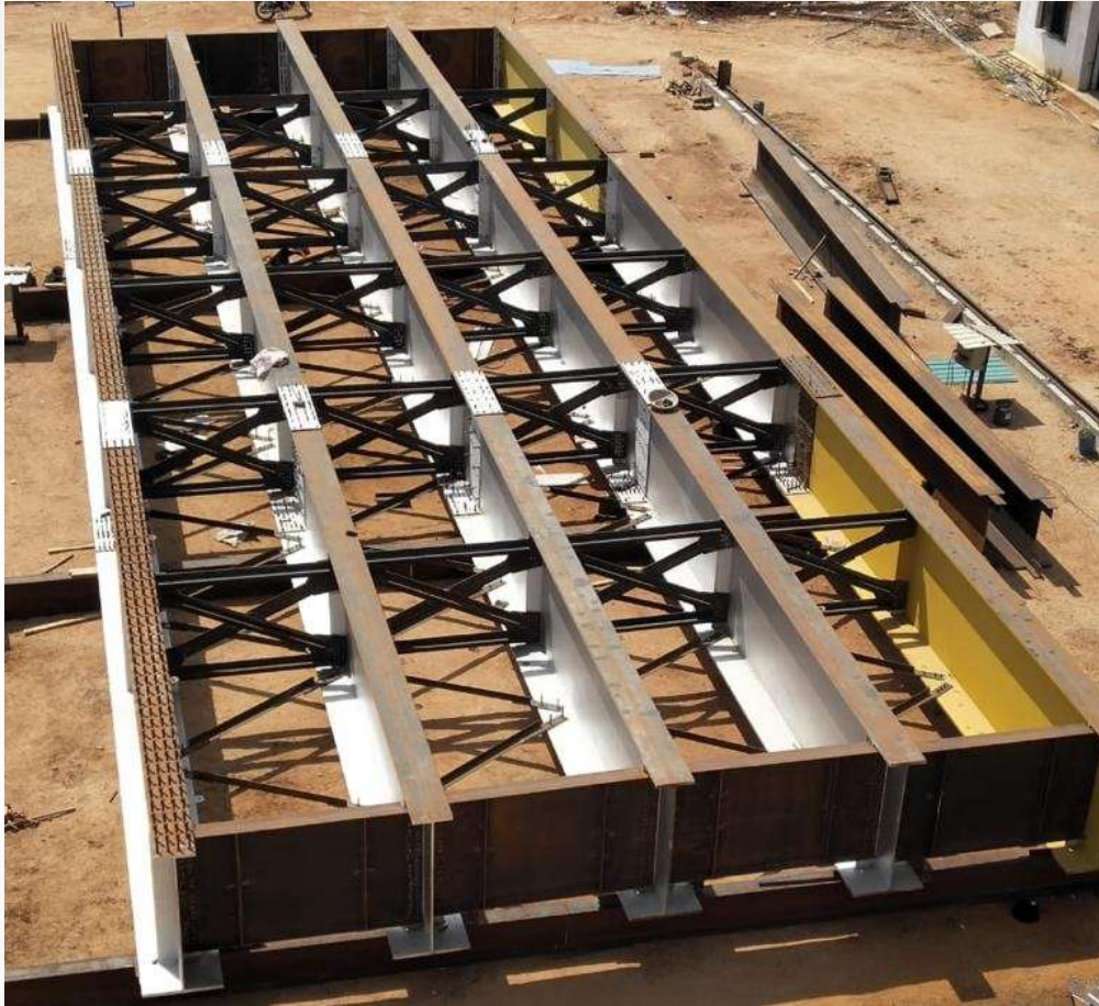
TRIAL ASSEMBLY OF 30.0M SPAN ROB
