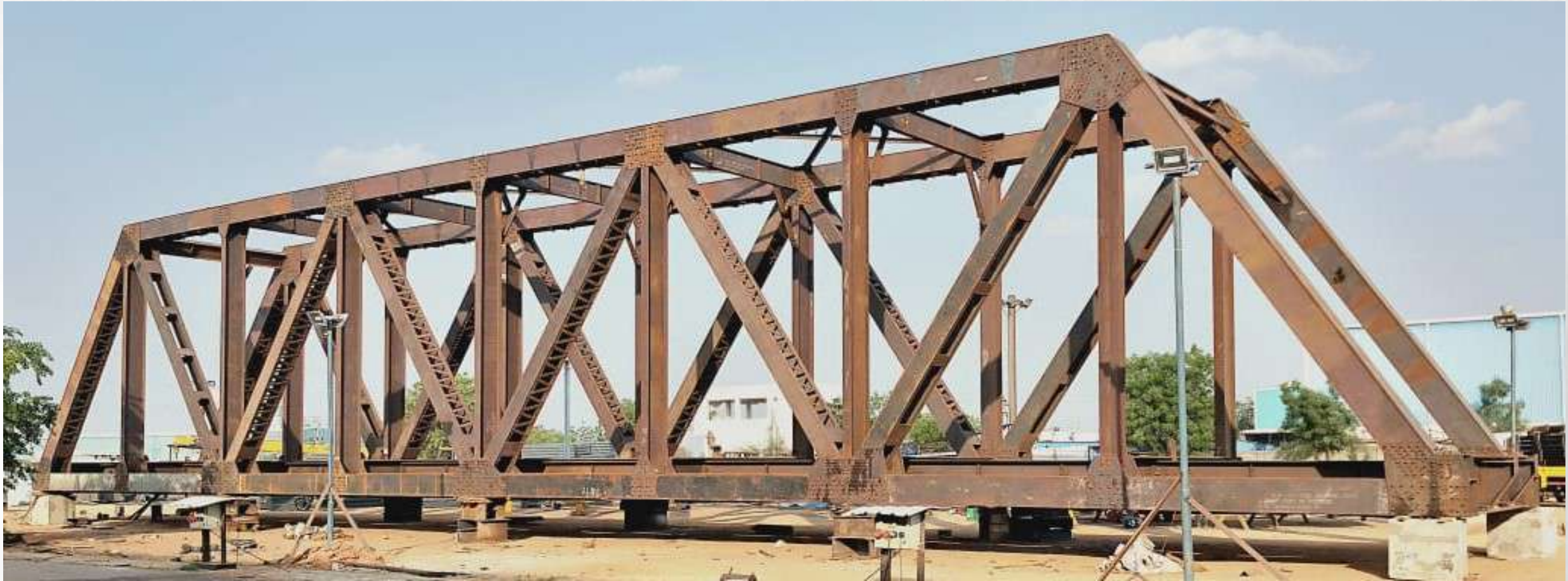
40.0M SPAN OPEN WEB GIRDER – BRIDGE NO-EAK213 - KERALA
