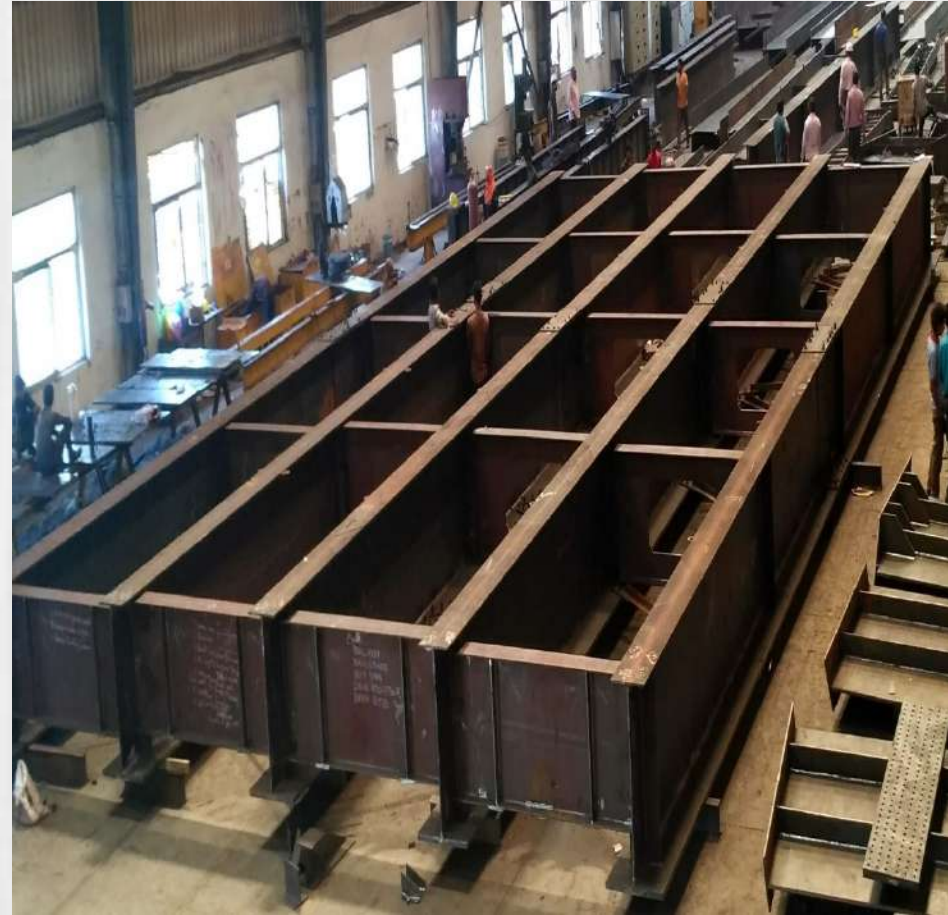
TRIAL ASSEMBLY 18.0M SPAN ROB
