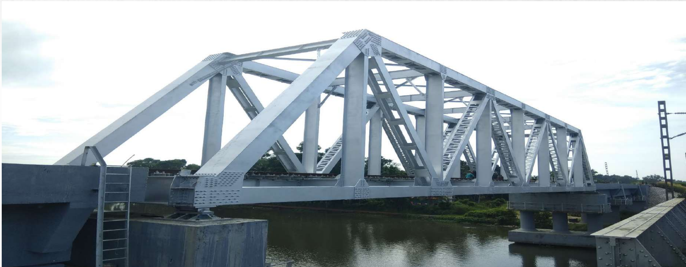
40.0M SPAN OPEN WEB GIRDER, KERALA
