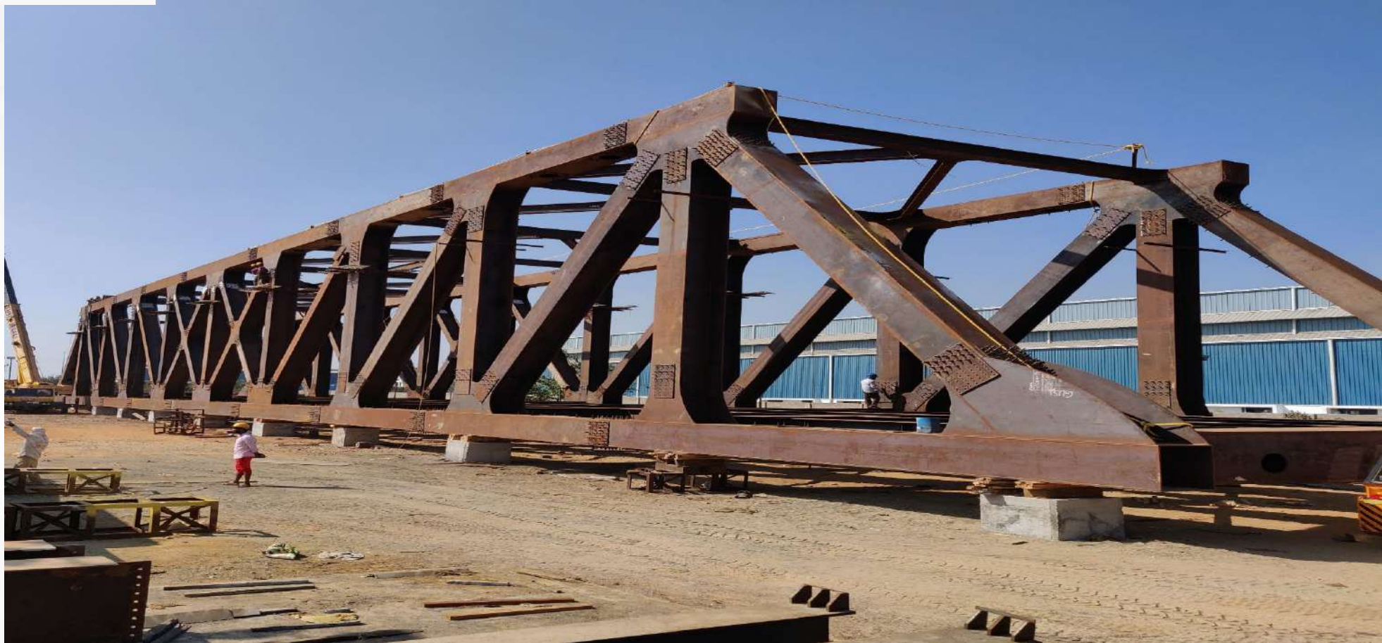
76.60M SPAN OPEN WEB GIRDER – PATRIPOOL KALYAN - MSRDC
